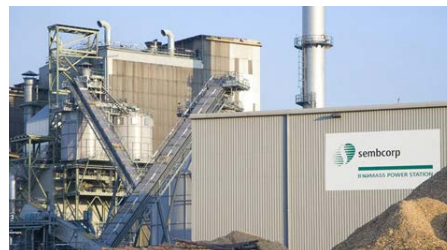
Wilton Location: Middlesbrough, England Customer: SembCorp Utilities (UK) Limited Start-Up Year: 2007 Capacity: 31 MWe Fuel: Short Rotation Coppice (SRC)
