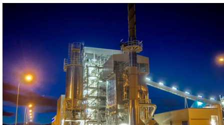
Biomass de cantabria at Reocin Location: Reocin, Torrelavega, Spain Customer: Ingeteam Power Plants, S.A. Start-Up Year: 2012 Capacity: 10 MWe Fuel: Biomass
